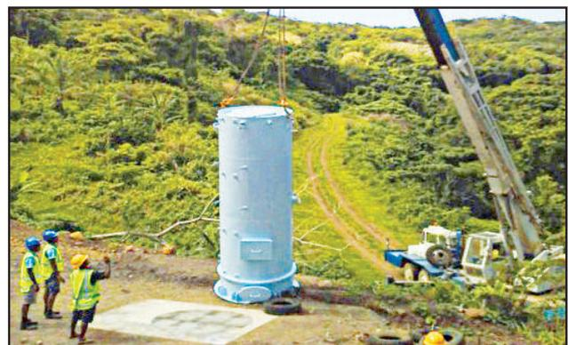
Installing the new Automatic Valveless Gravity Filter at Nabouwalu.
