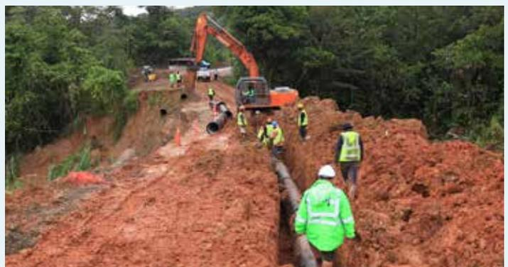
There is an important need to upgrade the water distribution system. Here WAF employees work around the clock to repair the trunk lines washed away by a landslide.
